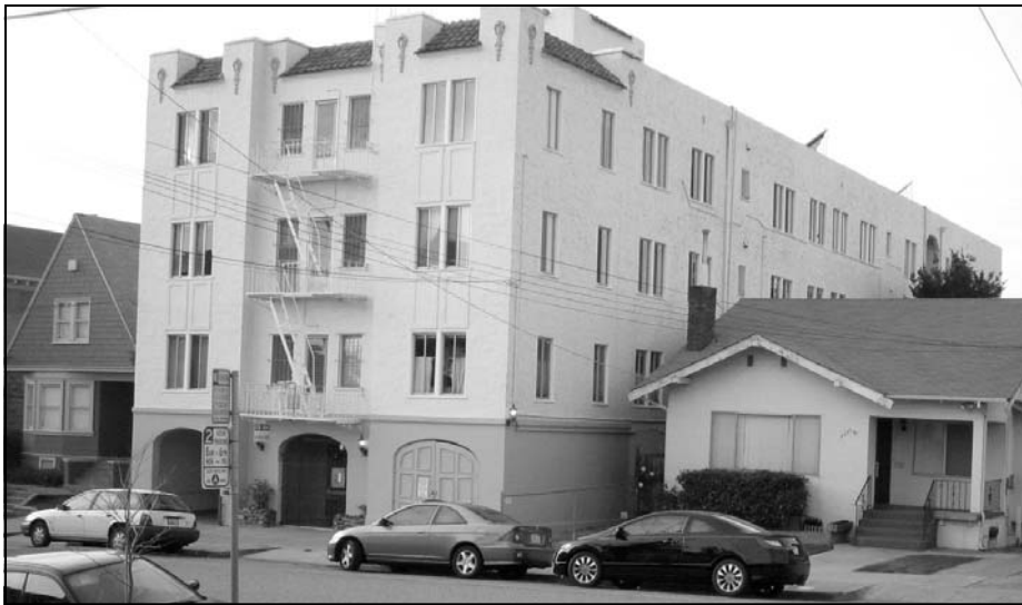
Zoning codes set the rules for height, density and uses on a property. These Montgomery Street buildings predate Oakland's current zoning codes, but new proposals may again allow mismatches of scale and density. See details in the article on page 1.
